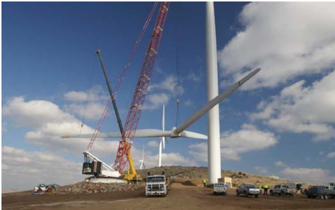
Figure 20 Turbine Construction, Woodlawn Wind Farm, Bungendore, NSW
