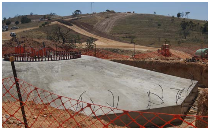
Figure 19 Turbine Base Construction, Woodlawn Wind Farm, Bungendore, NSW 26
