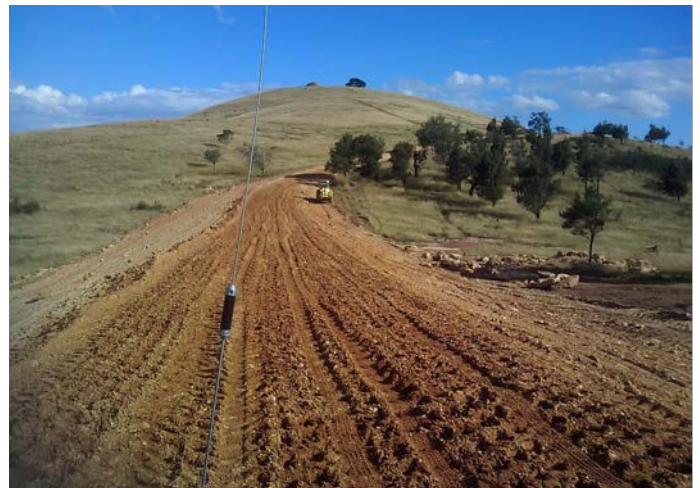
Figure 17 Road construction, Woodlawn Wind Farm, Bungendore, NSW 24
