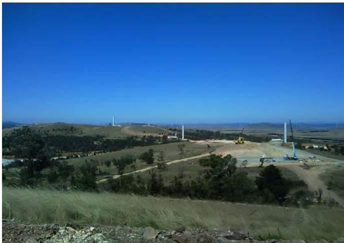
Figure 16 Construction of Woodlawn Wind Farm, Bungendore, NSW 23
