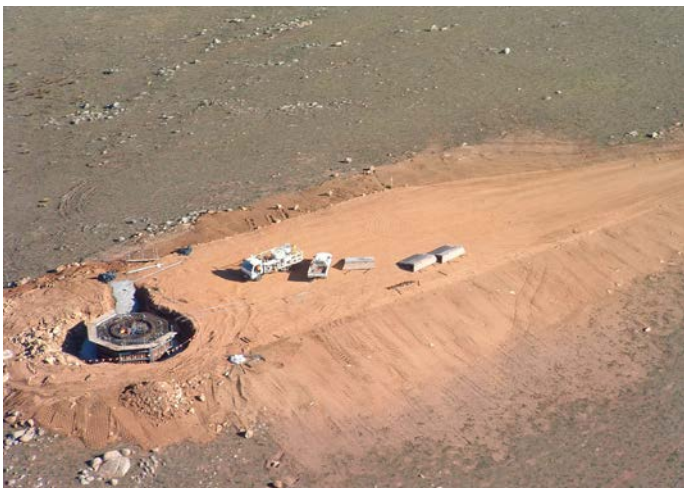
Figure 18 Turbine Base Construction, Woodlawn Wind Farm, Bungendore, NSW 25
