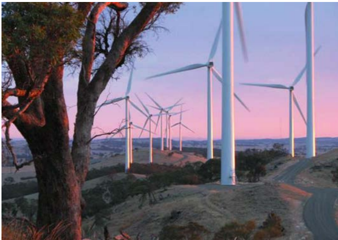
Figure 22 Sunset at Waterloo Wind Farm, SA 29
