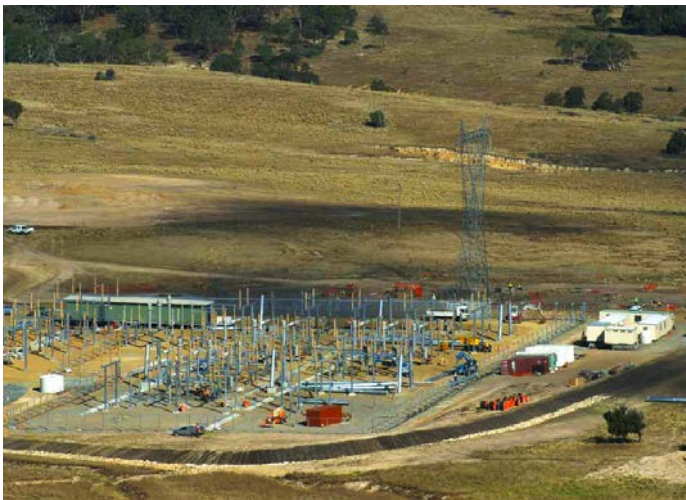
Figure 8 Building of substation, Bungendore, NSW 9
