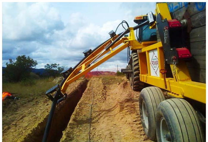
Figure 9 Laying cable, Bungendore, NSW 10
