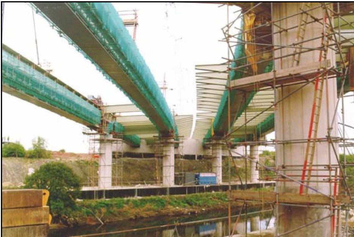
Exhibit 3.13 Aire Valley Viaduct under Construction
