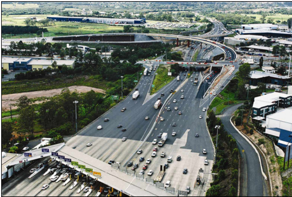
Exhibit 4.19 Port of Brisbane Motorway
