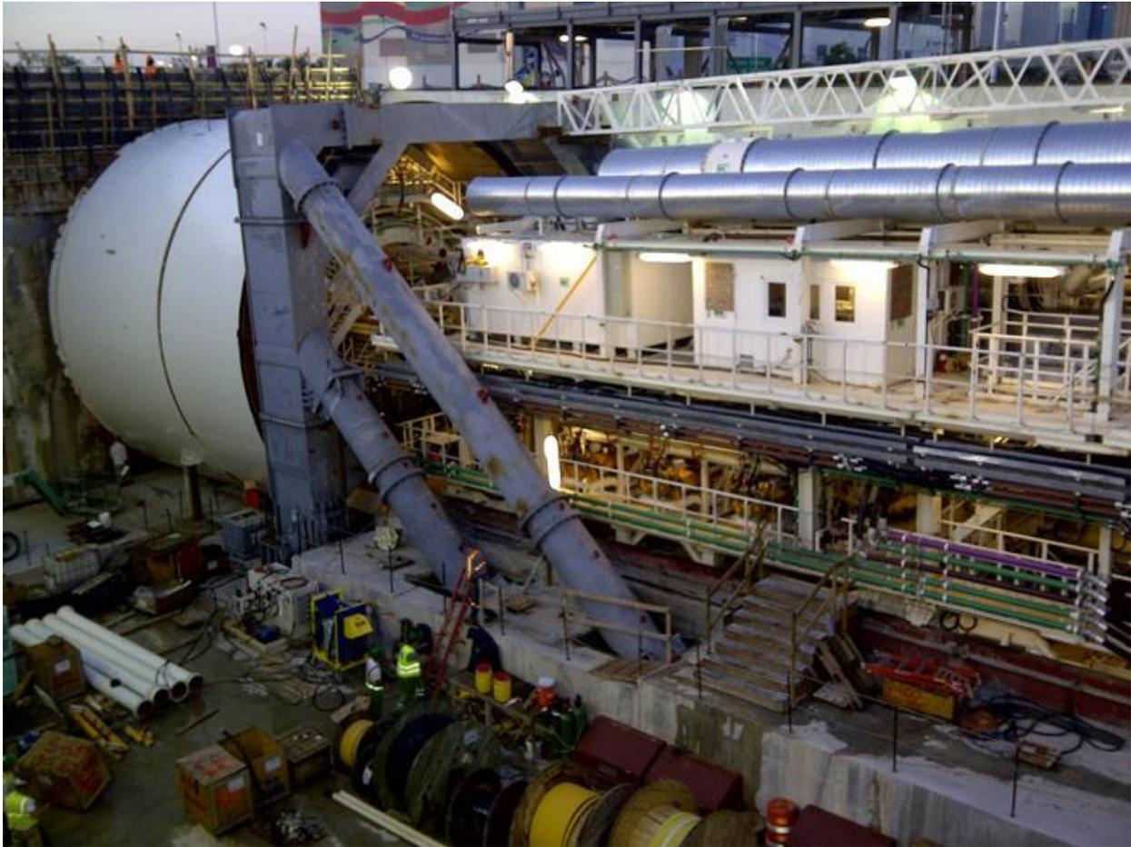
*The Tunnel Boring Machine trailing gear (credit: portofmiamitunnel.com)*
