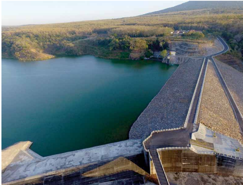
Bajulmati Dam, Jawa Timur Province
