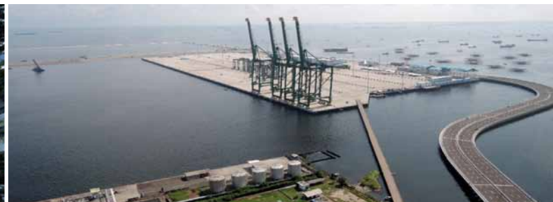
KALIBARU CONTAINER TERMINAL 1. The largest port in Indonesia. Awarded by the Asian Civil Engineering Coordinating Council
