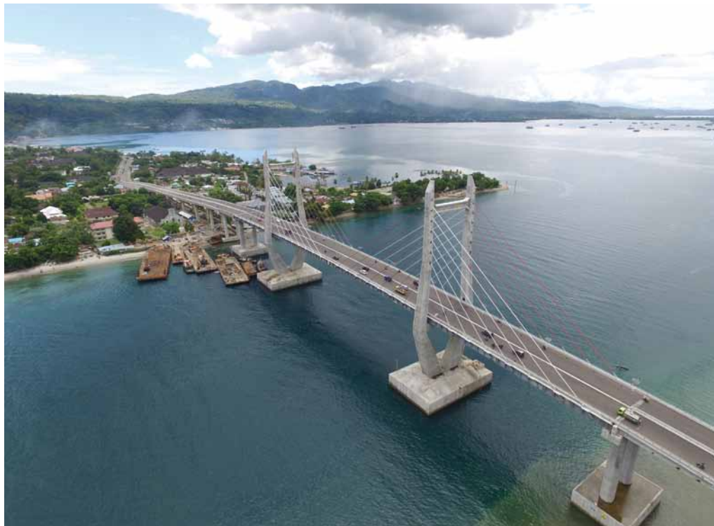
A bridge constructed in Maluku Province
