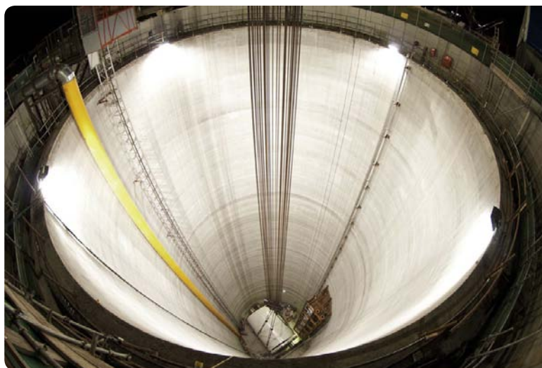
Image courtesy of Thames Tideway Tunnel ( www.tideway.london )
