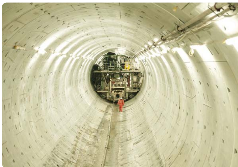
Image courtesy of Thames Tideway Tunnel ( www.tideway.london )
