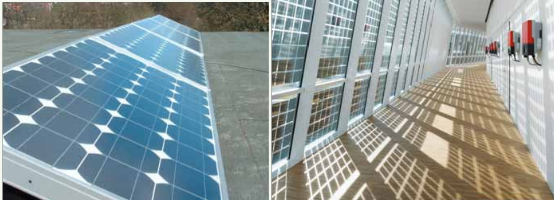
Figure 35: BAPV (Left) and BIPV (Right) Systems
