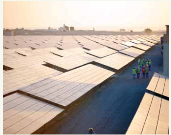
Figure 21: O&M Workers at a Large-scale Solar PV Power Plant
