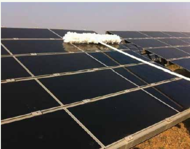
Figure 26 : Module Cleaning Using Dust Broom
