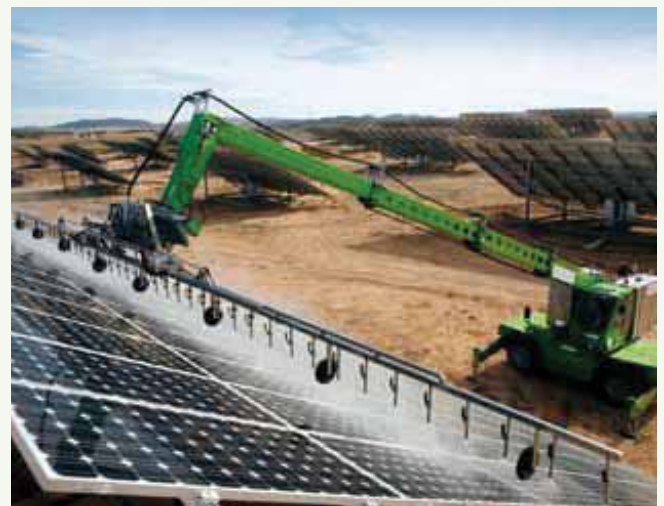
Figure 24: Module Cleaning Using Crane
