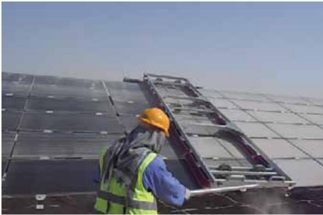
Figure 25: Module Cleaning Using Brush Trolley
