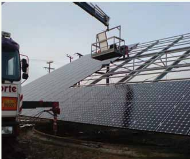
Figure 23: Module Installation on a Large Tracking System
