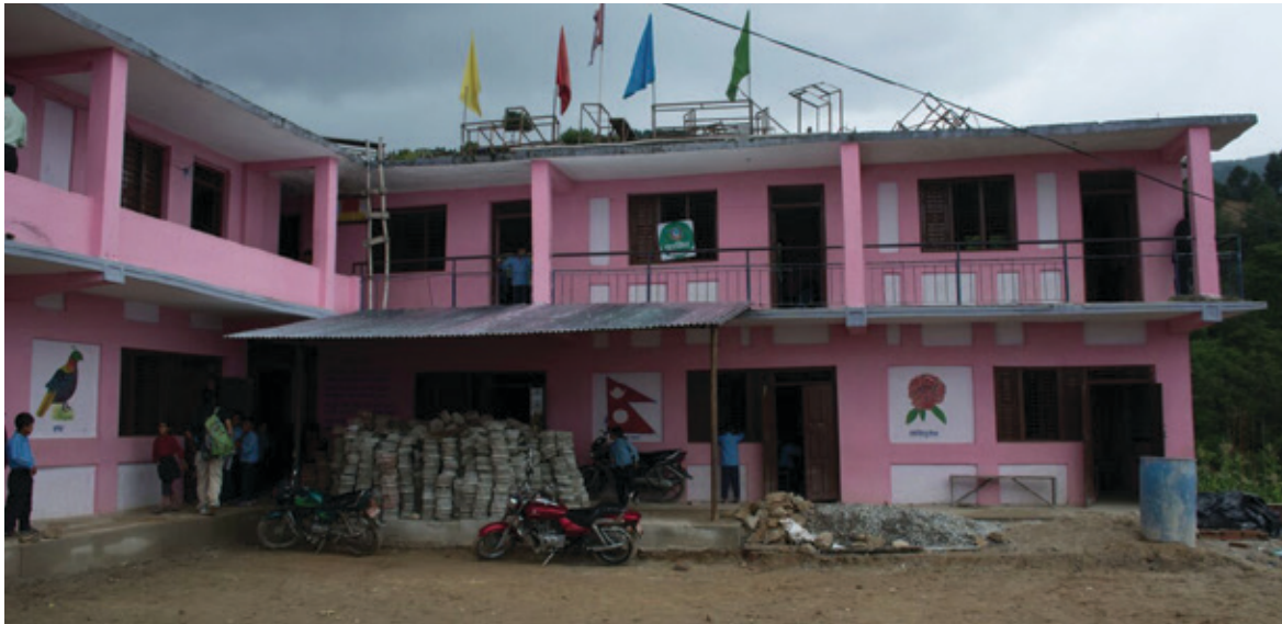
Successfully retrofitted school buildings that were undamaged in the earthquake.
