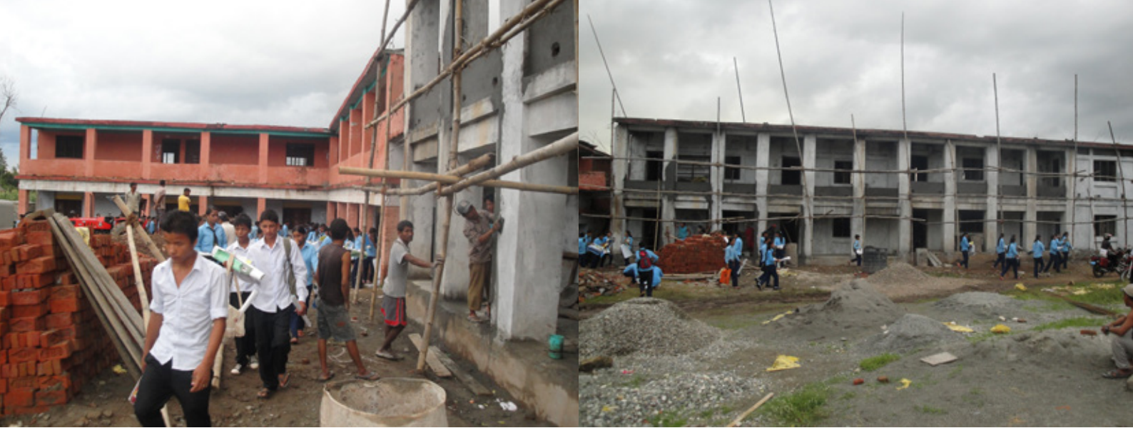
Schools undergoing retrofitting in Dhangadi before the earthquake.
