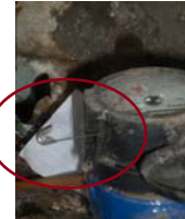
Water meter removed and replaced with straight pipe.
