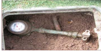
Pipe used to partially bypass water meter.
