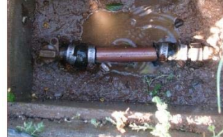
Water meter removed and replaced with straight pipe.
