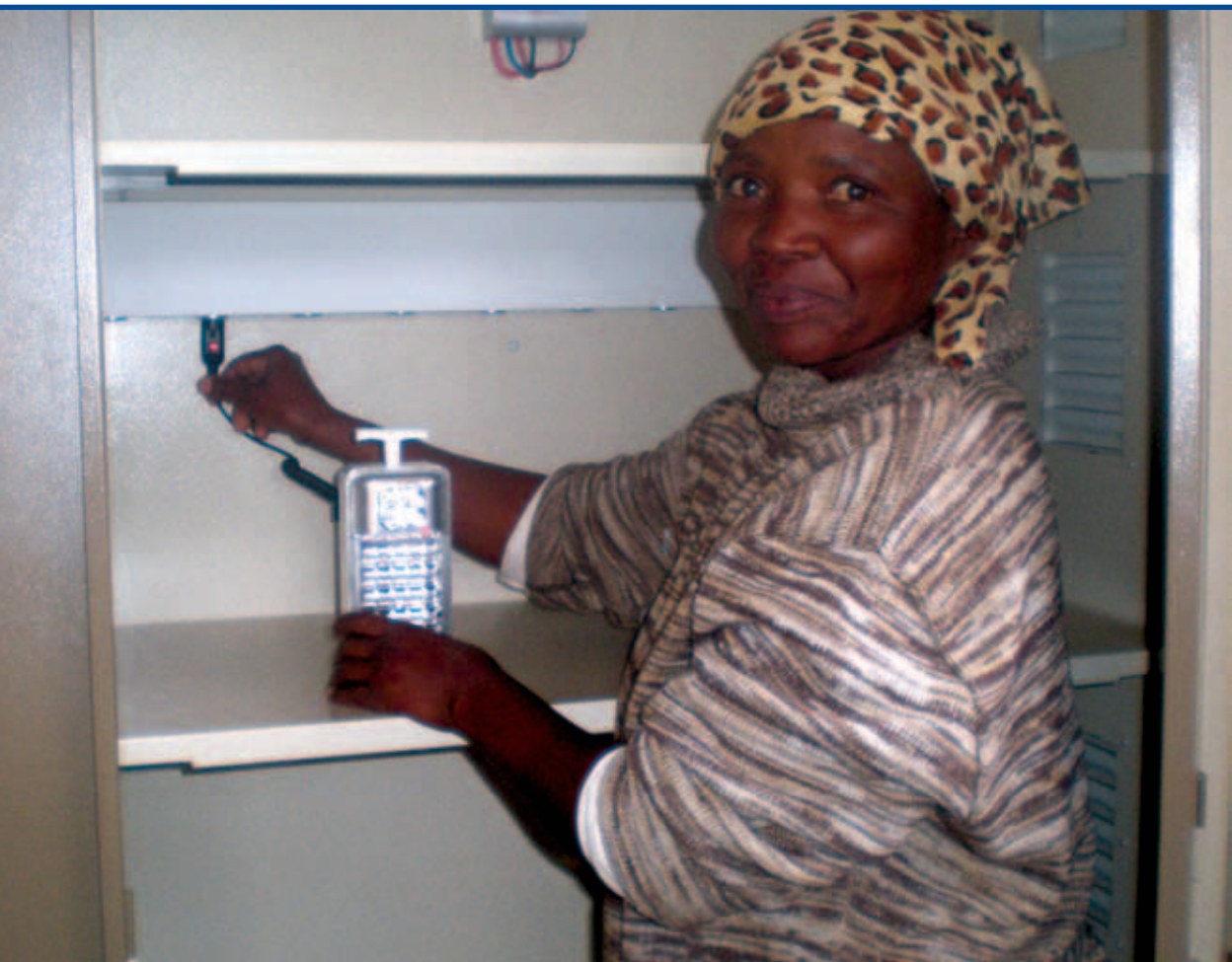
Woman in Botswana showing her Ready-Box, a ready to use house wiring box, reducing the cost of wiring a house
