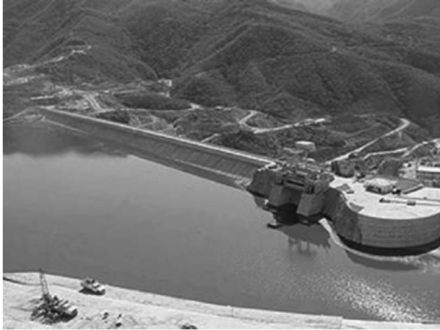
Figure 11. A Photograph of the Dam and the Powerhouse, Mexico
