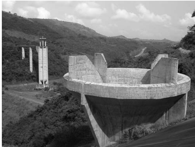
Figure 5. View of the Morning Glory Spillway of the Bumbuna Hydroelectric Project, Sierra Leone
