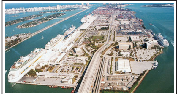
Port of Miami Tunnel, Florida (DBFO with availability payments). Expected to open in 2014, the tunnel will connect the Port of Miami with the MacArthur Causeway and I-395. Senior bank debt, a TIFIA loan and private equity have been used to finance the project. (Photo: FHWA)
