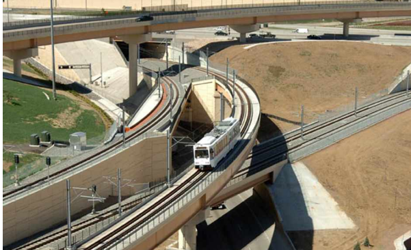
Location: Denver, Colorado
