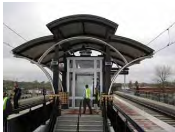
Attractive architectural station design in Charlotte, North Carolina, USA. Photo by and reproduced by kind permission of James Dwyer.
