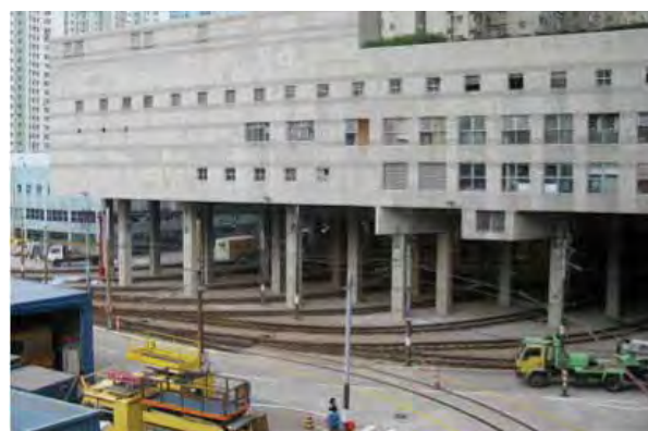
Hong Kong, China. The Tuen Mun LRT has exploited air rights development over its depot. Photo by and reproduced by kind permission of Scott McIntosh.
