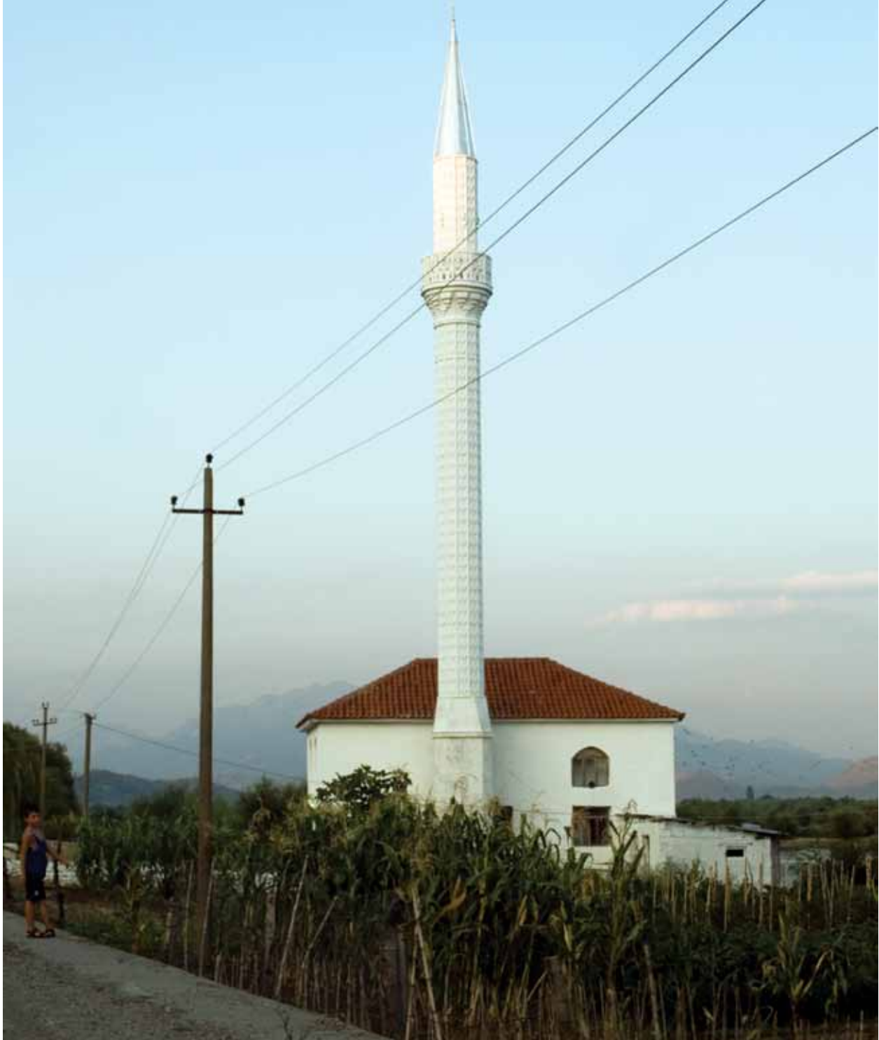
Power lines bring electricity to rural areas of Albania.
