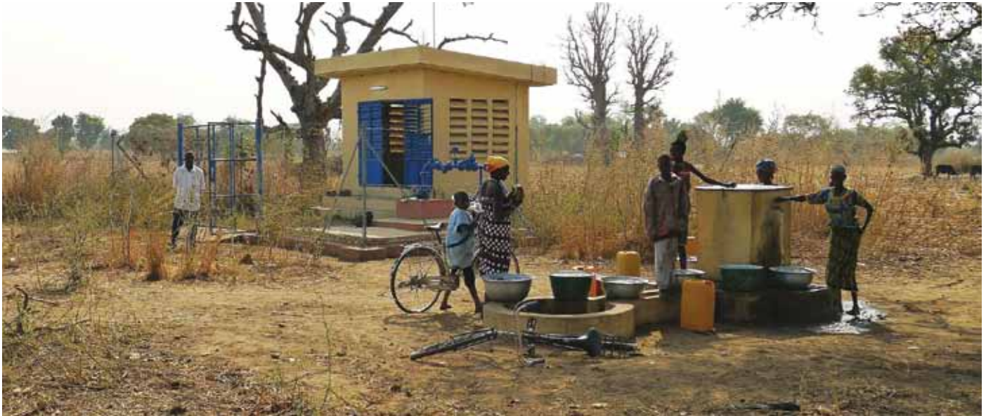
Sustaining coverage and improved access in rural and small towns.
