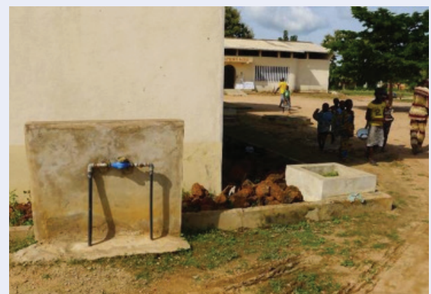
Household connection in the village of OUNET, Municipality of Banikoara, Department of Alibori, Benin. (Photo by Fichtner)
